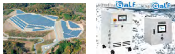
Mega solar business that provides one stop services ranging from system design to construction and maintenance
