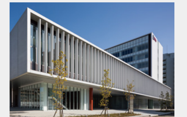
IDEC Head Office / Technology Research Center
