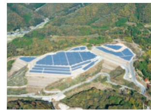
Sayo IDEC Solar Power Station
