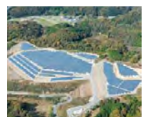
Mega-solar power business
